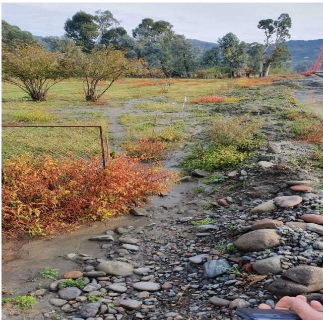
Flooded land plot adjacent to stone column construction site
