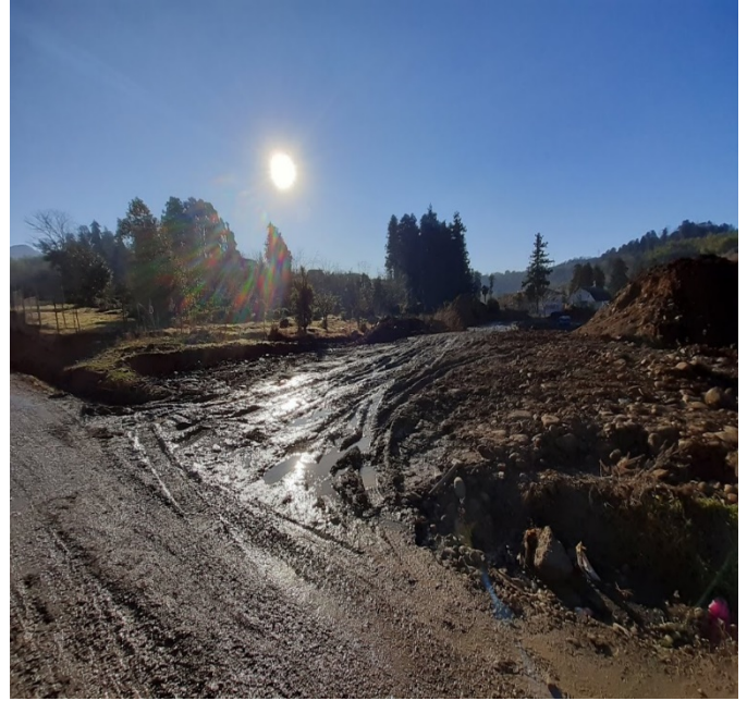
Local road intersecting with access road to Bridge N3
